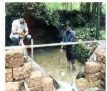
Fig. 1.1.7.6 Construction of a v-notch
