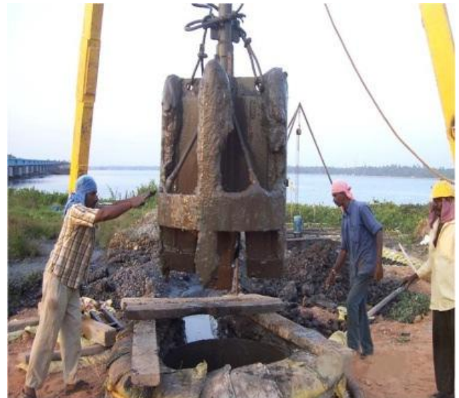
Fig 2.8.2 Drilling of bore holes by CMRL in progress
