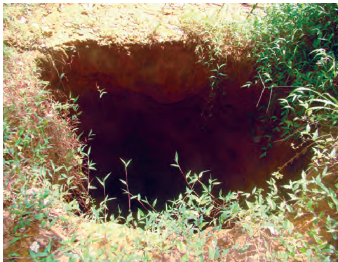
Fig. 2.1.1.1 View of the collapsed surface
