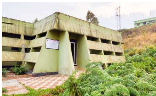
Fig. 1.9.5.2: GEObs initiated in the State Police Department building at Sankhumalai, Munnar.
