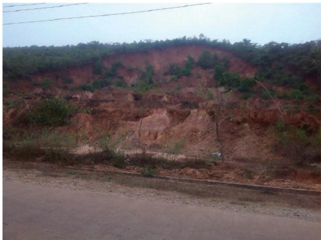
Fig. 1.11.1 A distant view of slope failure initiated in the lithomargic clay at the base of a deep laterite profile at Kadwad near Karwar.
