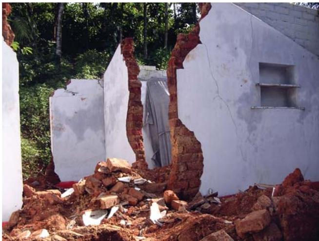
Fig. 2.1.1.4. A house completely damaged in land subsidence in Kunnamangalam Vayal
