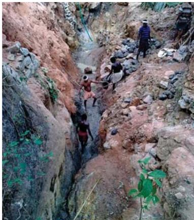
Fig.3.1.1.1 Construction of sub-surface dyke in progress in Paramkode watershed
