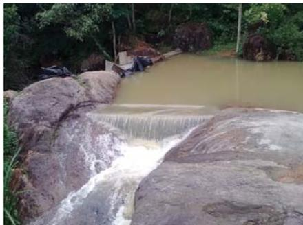
Fig. 3.1.1.2 Check dam at Erappupara in Peruwanthode watershed
